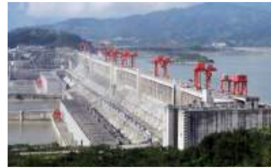
Three gorges dam (China)
